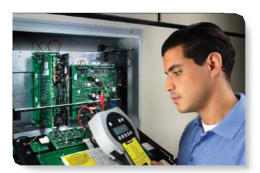
The Simplex 4100ES (eServices) Fire Alarm Control Panel is a premier fire detection and alarm system. Built upon the legendary, field proven performance of the Simplex 4100U Series the next generation 4100ES leverages new technology, design improvements, T-Tap wiring and IP-based diagnostics to offer low cost installation that electrical contractors can appreciate.
